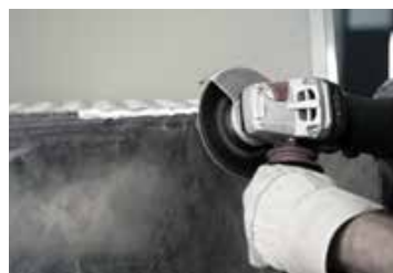
Removing welded seams
